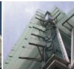
APECBC Headquarters, Richmond – steel structure and steel supported shading
