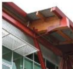
National Works Yard, Vancouver, LEED Gold
