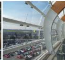
Brentwood Skytrain Station, Vancouver, Busby Perkins and Will
