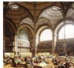
Bibliothèque Nationale, Henri Labrouste - early cast iron and modular construction
